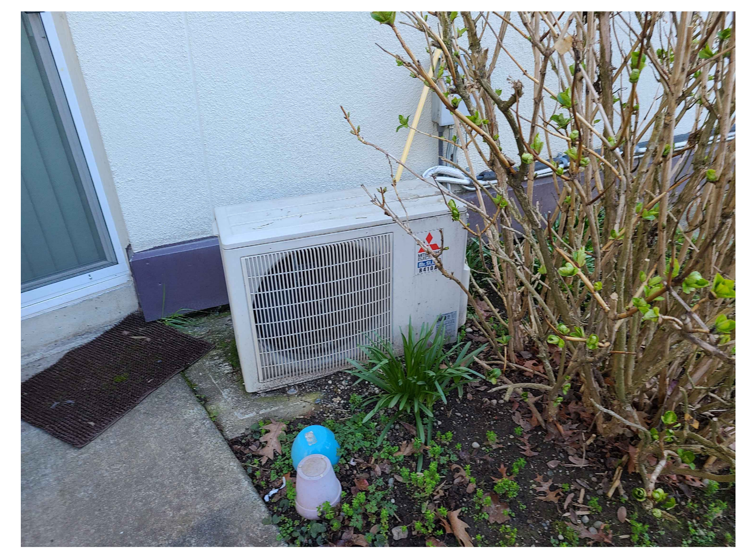
EXISTING AC CONDENSER C NTS M0-1
