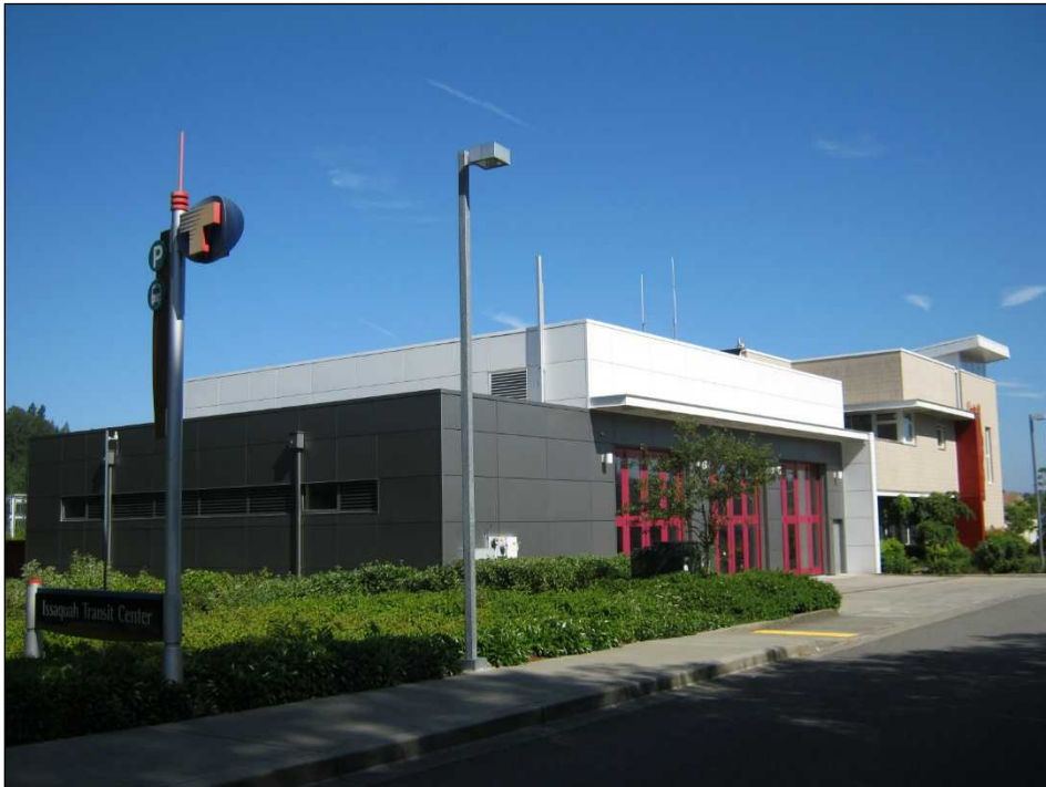
23. Adjacent fire station to the west
