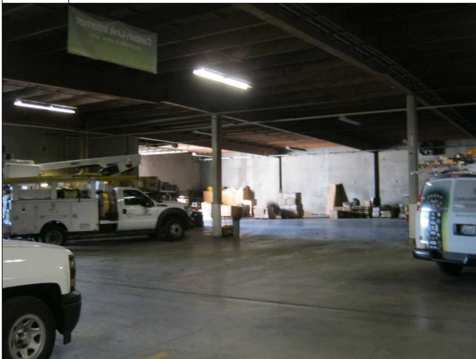
20. Interior garage area with floor trench drain
