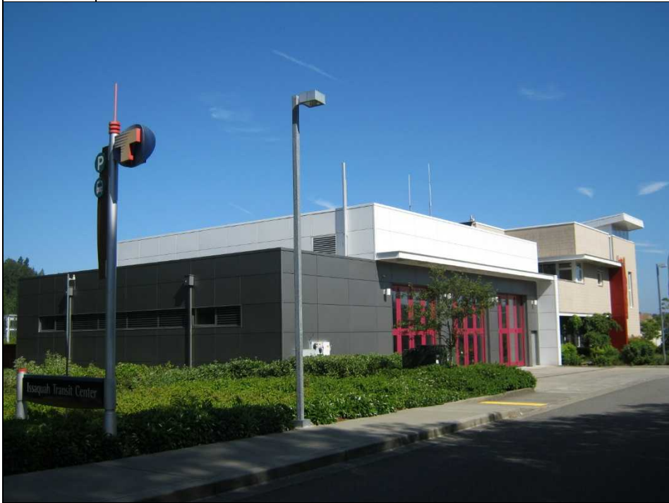
10. Adjacent fire station to the west
