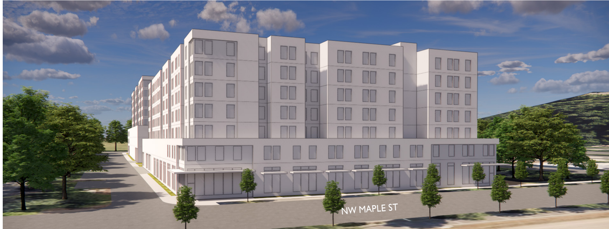
NORTHEAST MID LEVEL VIEW
