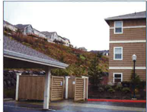
This dumpster enclosure is located out of the line of sight and away from walkways.
