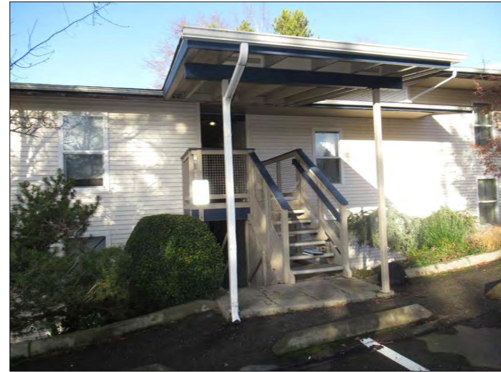
EXTERIOR STAIR AT BUILDING 'O' (BUILDING 'Q' IS SIMILAR)
