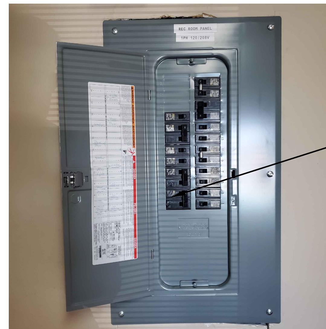
2 PHOTO 2 - TYPICAL REPLACEMENT LOAD CENTER NTS
