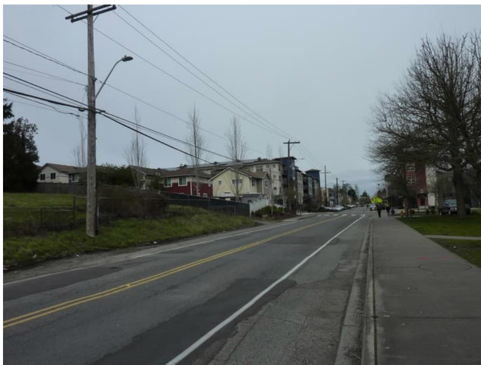
Looking north along 8 th Avenue SW, with the west subject parcels on the left.
