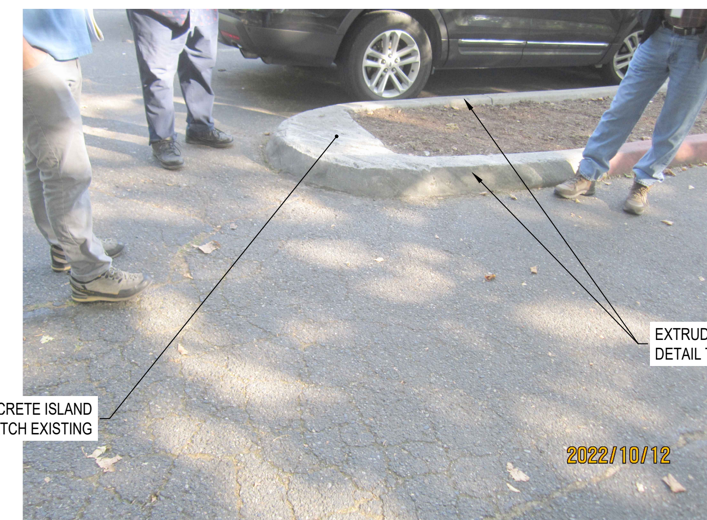
205 C01 CONCRETE ISLAND REPLACEMENT NOT TO SCALE
